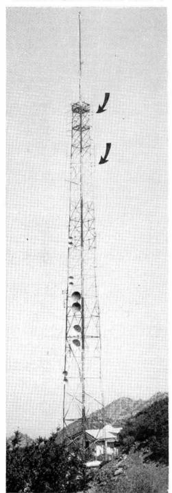
TWO SANDIA RADIO ANTENNAS are among the 50 positioned on this 225-ft. tower atop Mt. Diablo. Upper arrow points to the Sandia antenna for transmitting; the lower arrow, the antenna for receiving.
